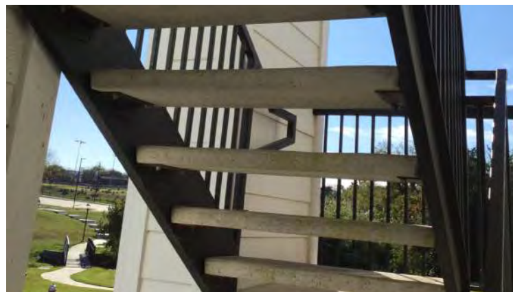
Photos of general site/ accessibility
