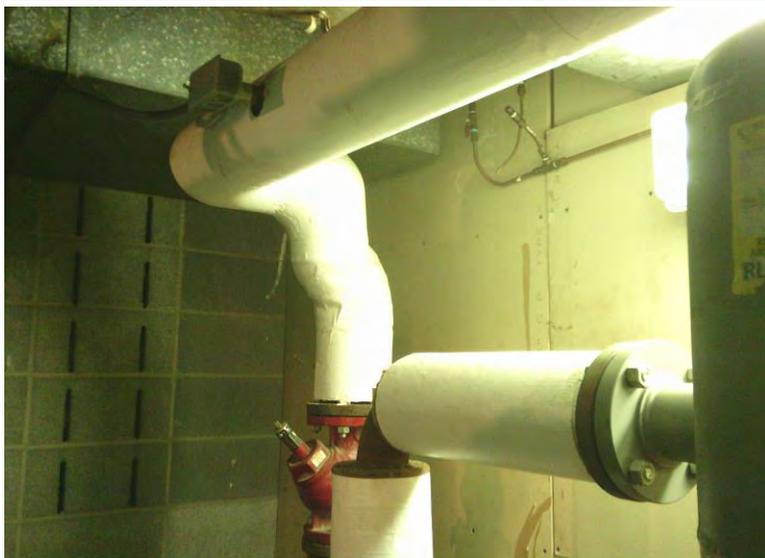
**18. Asbestos Homogeneous Area 9 – Newer fiberglass pipe insulation runs with white mastic and foil paper covering; Samples 13 through 15**
