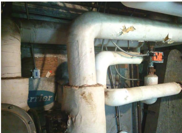
15. **Another view of Asbestos Homogeneous Area 7 – Foam insulation elbows and fittings with canvas wrap and white mastic; Samples 07 through 09**
