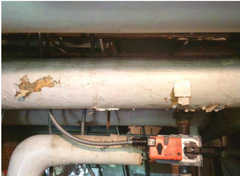
**16. Asbestos Homogeneous Area 8 – Older fiberglass pipe insulation runs with white mastic / wrap and foil paper covering; Samples 10 through 12**
