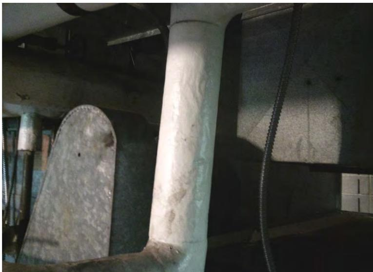
**17. Another view of Asbestos Homogeneous Area 8 – Older fiberglass pipe insulation runs with white mastic / wrap and foil paper covering; Samples 10 through 12**
