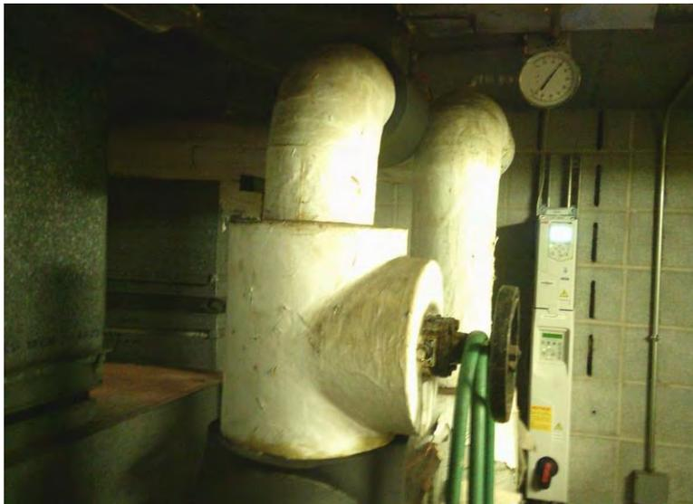
14. **Asbestos Homogeneous Area 7 – Foam insulation elbows and fittings with canvas wrap and white mastic; Samples 07 through 09**
